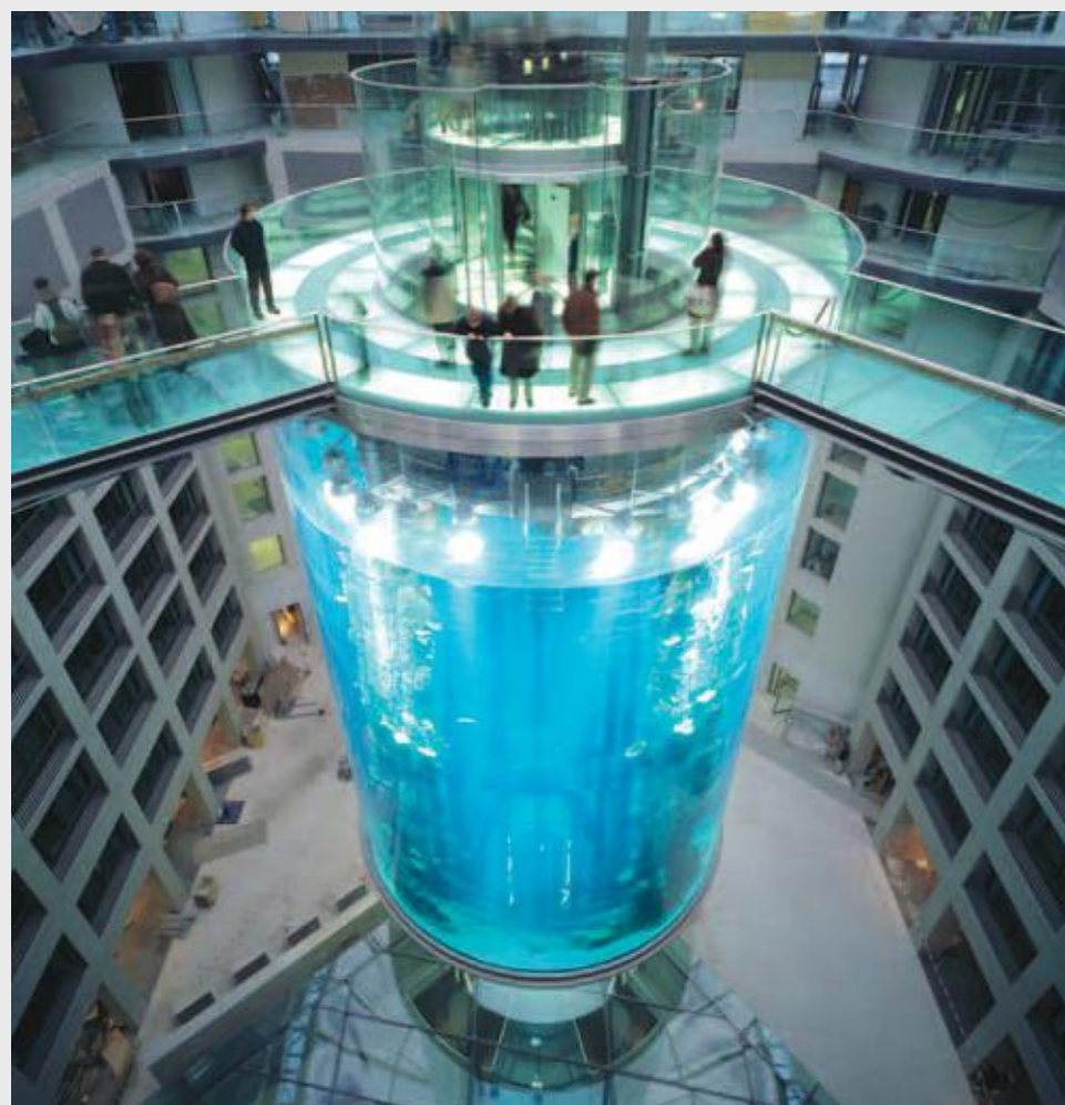
MMA was the raw material for this ground-breaking aquarium, which forms the centrepiece of Berlin's DomAquaree hotel and leisure complex. Suspended 8 m off the ground, the cylindrical aquarium is made from 150 tonnes of high-optical clarity acrylic. A seven-minute narrated elevator ride through the structure allows a good view of more than 2,500 fish swimming in the one million litre artificial seascape © Christian Gahl
